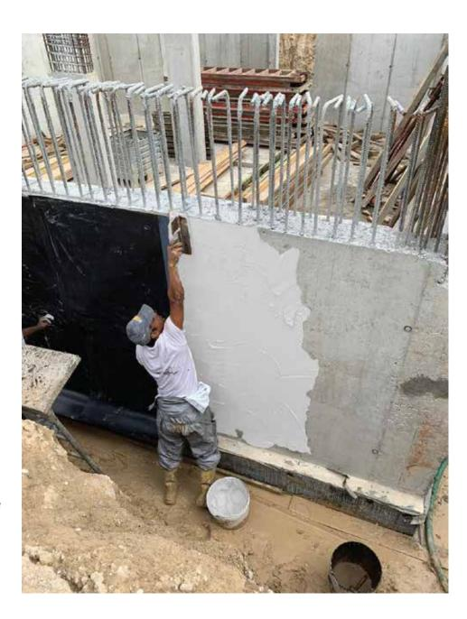
**The self-priming cement-based adhesive, SikaShield® W1,** acts as levelling compound and a sealing adhesive resulting in a strong and lasting bond between the concrete substrate and the membrane, avoiding any lateral water migration and reducing the risks of leakages.
